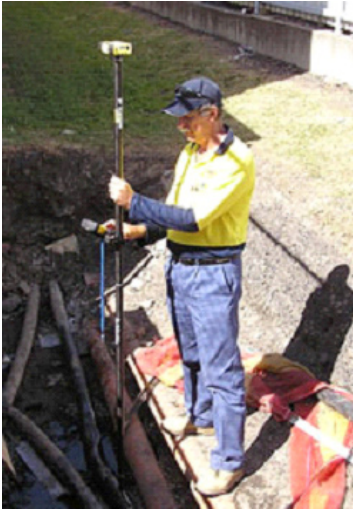
GPS being used to capture the position of a new joint.
